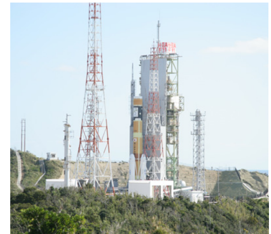
Cryogenic Test Nov. 9, 2006
